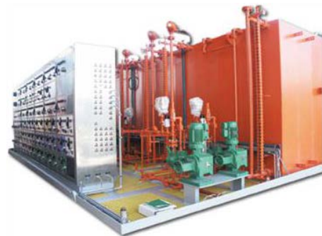
Chemical Injection Packages Customer: Petrobras
