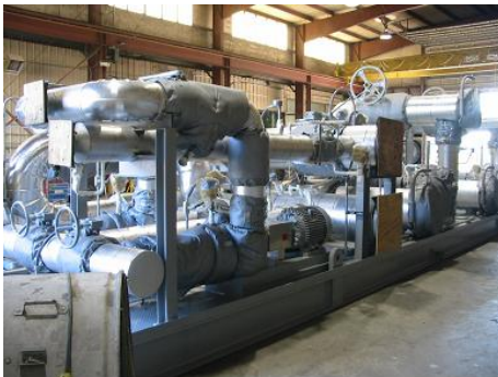
Intercooler Water Circ. Package Customer: GE/Basin Electric
